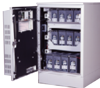
Radium MiniBay XRT with alarmed battery breakers
